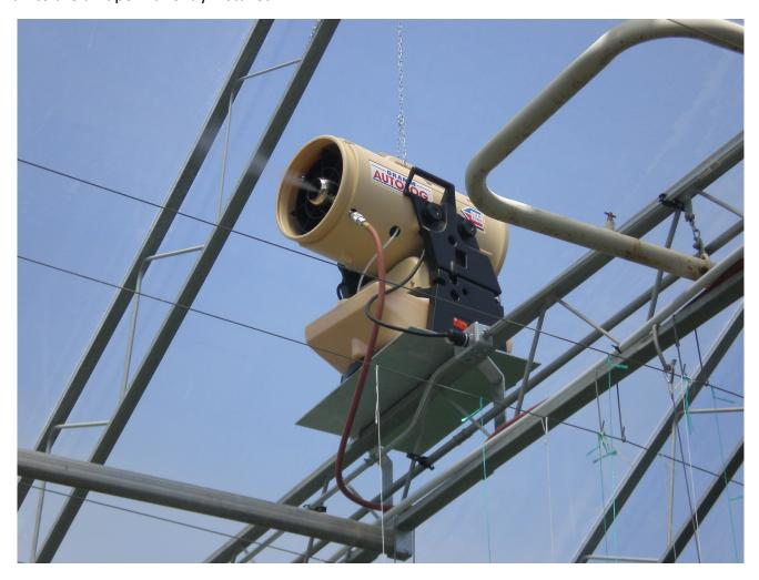
To be operated, each Autofog head will require two control circuits: one 24 VAC for the air valve to control the fog and one line voltage to operate the fan and agitation.
